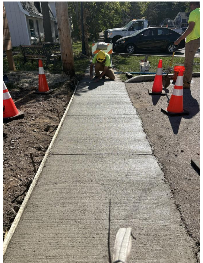
Repairing sidewalks downtown in-house
